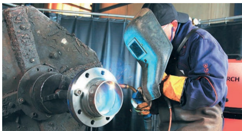
Luis Braga welds the root layer of the pipe socket with a Lorch S-SpeedPulse machine using Lorch's SpeedRoot process. The top layer is welded with Lorch SpeedPulse.
